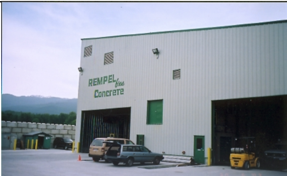
Completed Ready-Mix Plant at Rempel Bros. Concrete Ltd.'s North Vancouver facility.
