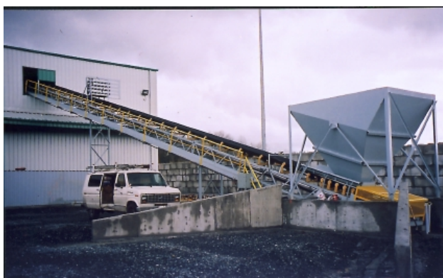
Installation of conveyor
