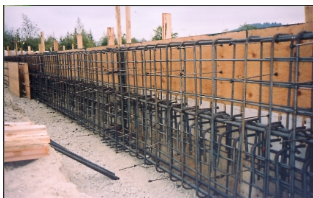
Reinforcement of perimeter beam
