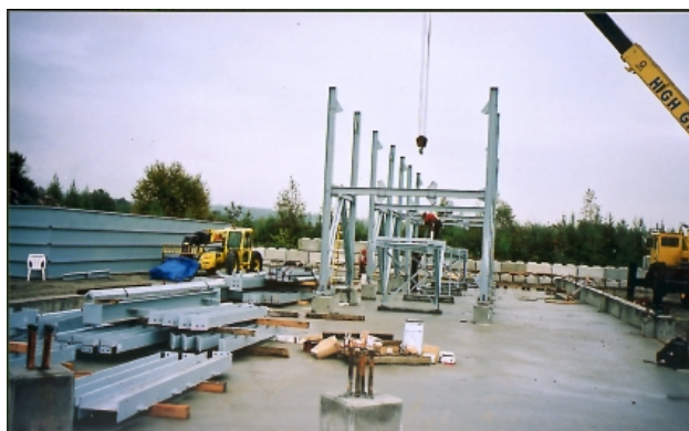
Installation of equipment
