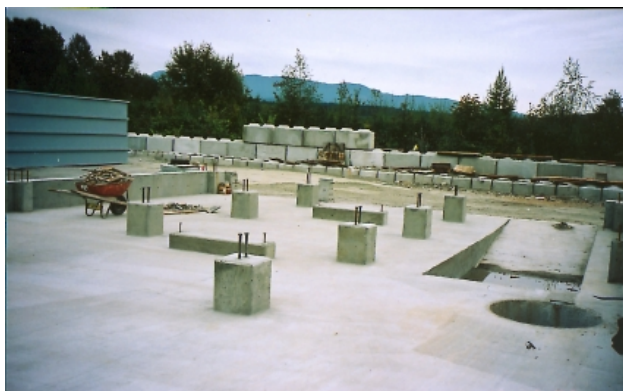
Completed slab with pedestals for equipment
