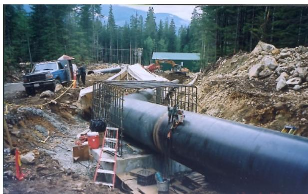
*Installation and welding of penstock. Construction of thrust block.*
