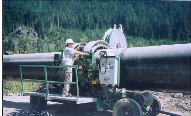
*Preparation and fusing of plastic pipes*
